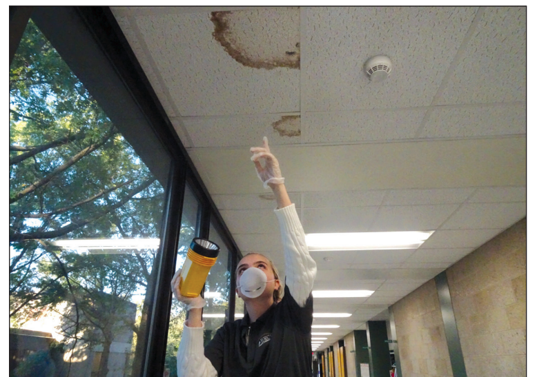
A visible water stain spreads across ceiling tiles in the MS building directly above hallway heating vents.
